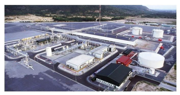
The Nam Con Son Onshore Gas Processing plant handles a gas rate of 370 mmscfd and liquid handling facilities for a peak rate of 5625 bpd of stabilised condensate.
