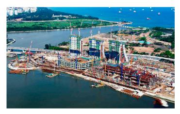
A design and construct contract for marine works as part of the 40 acre Marina Bay development in Singapore. The project was completed in 2010 and included a promenade deck, a purposebuilt 5,000 m<sup>2</sup>. Events Plaza superstructure, and two submerged concrete structures with underwater tunnels for a new retail concept called the Crystal Pavilions.
