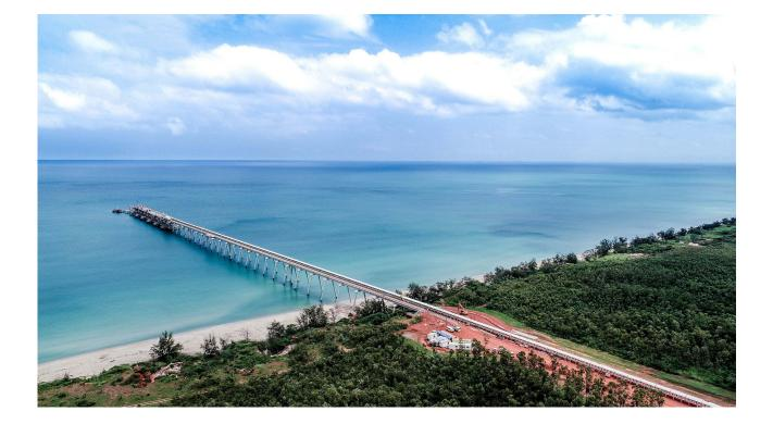
McConnell Dowell constructed a bauxite export facility with a 624 m jetty and a 299 m wharf in remote North Queensland. The scope also included the onshore construction of conveyor and transfer stations works linking into the reclaim conveyor. McConnell Dowell selfperformed much of the construction.
