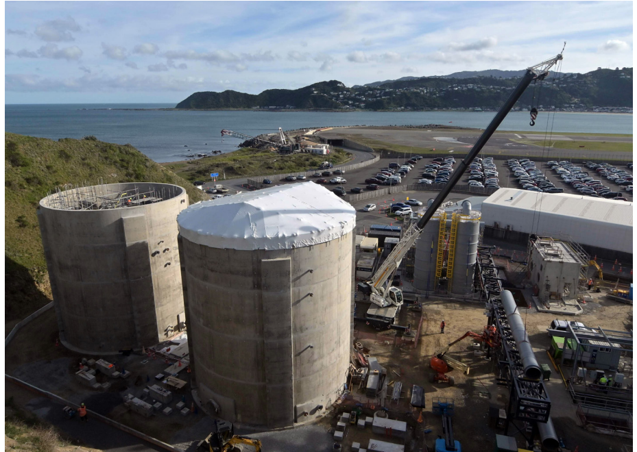
The first pipe (bottom right) is placed on top of the pre-assembled pipe bridge on 28 July
