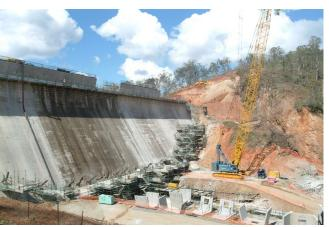
90,000M3 OF EARTHWORKS **69 POST TENSIONED GROUND ANCHORS INSTALLED DAM WALL RAISED BY 5.8M** WINNER QUEENSLAND CIVIL CONTRACTORS **FEDERATION EXCELLENCE AWARD**
